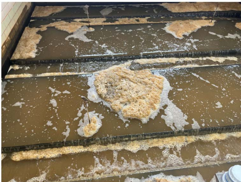
Filter Backwash Cycle
