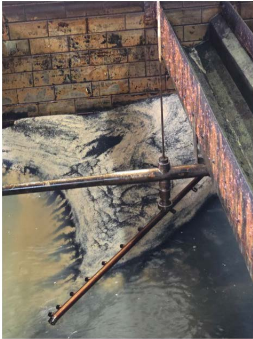
Ex. Drained Filter Basin (Drained, & Unbalanced Surface Wash )
