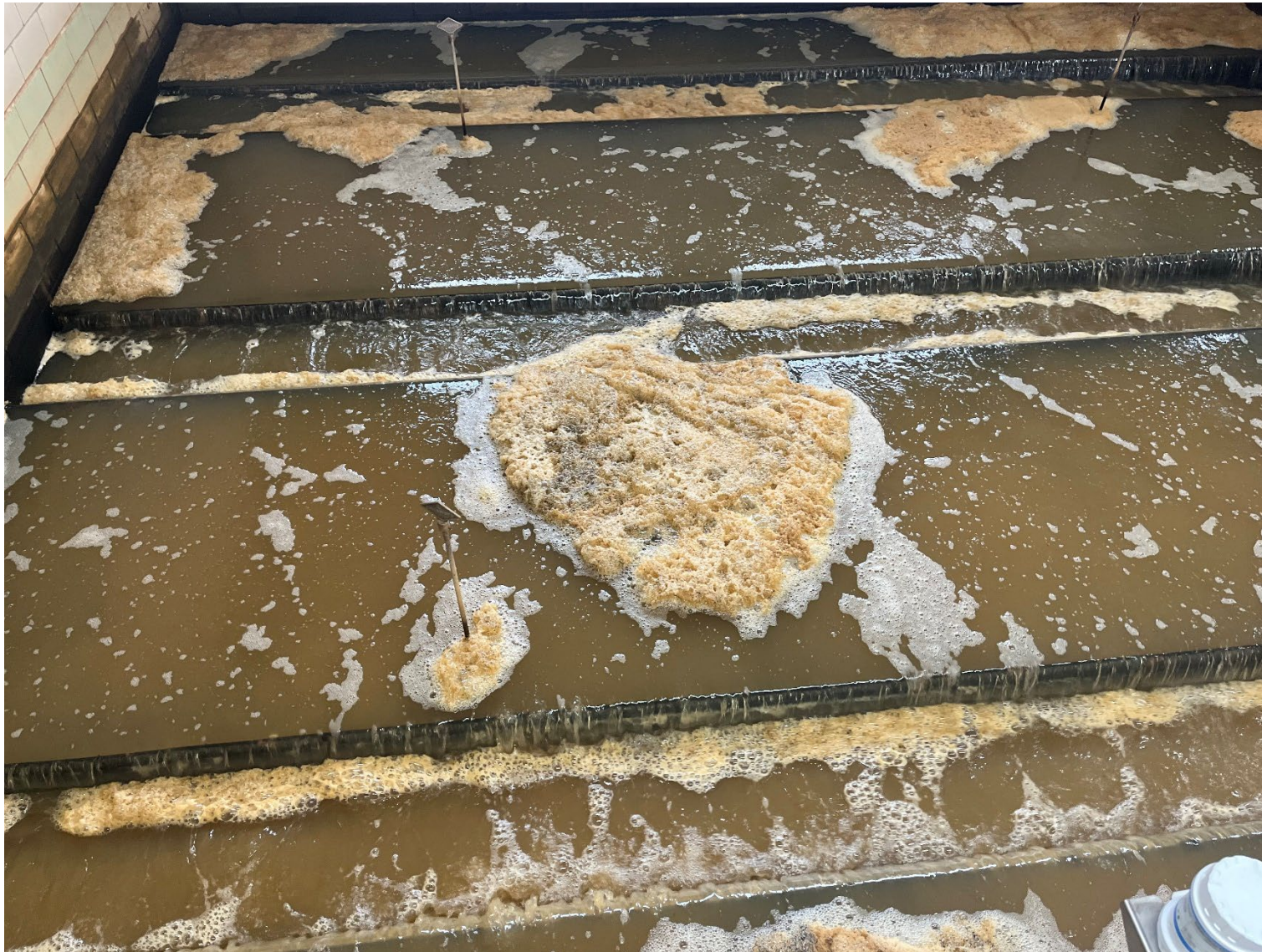
Filter Backwash Cycle
