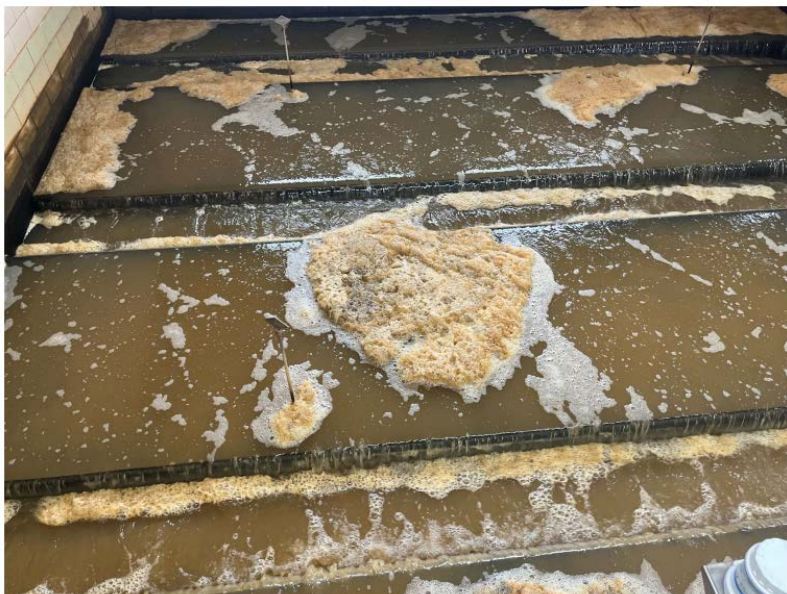
Filter Backwash Cycle
