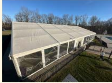
Exterior Roof Panels
