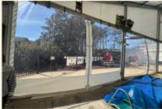
Recently Replaced Clear "Café" Panel
