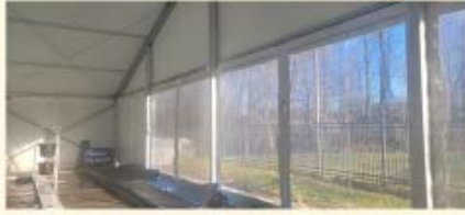
Clear Panels from Interior
