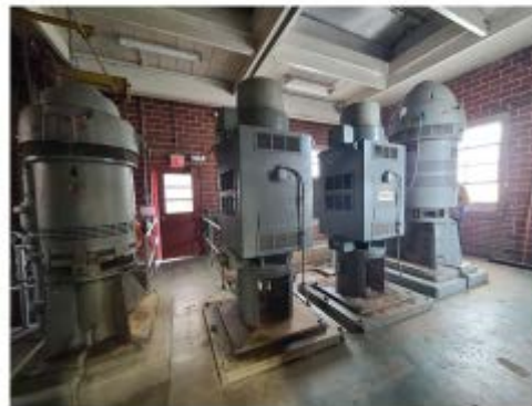
RAW WATER INTAKE PUMPS
