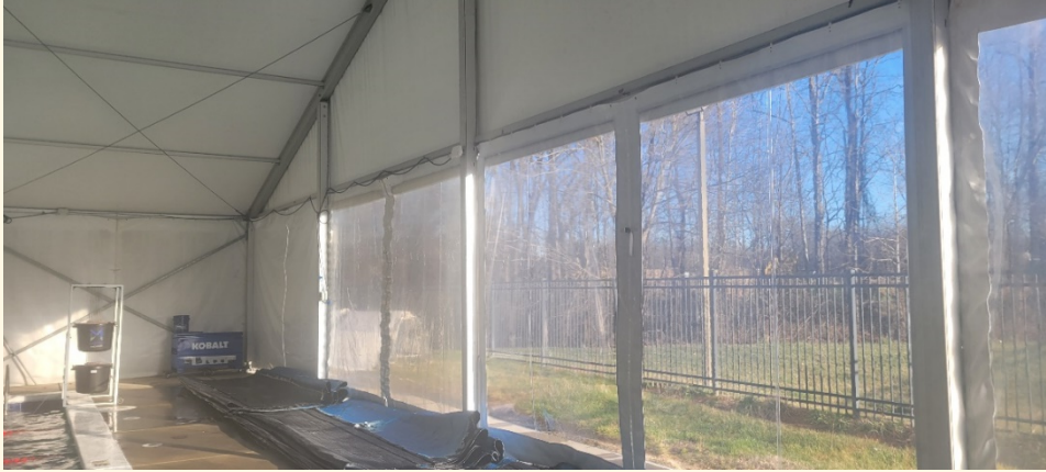
Clear Panels from Interior
