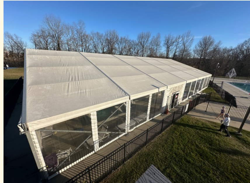
Exterior Roof Panels
