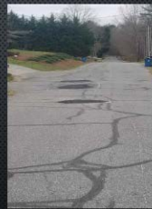
Pothole repair Mical Ave
