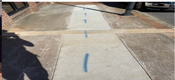
Front of WSVM facing East
