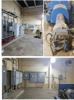
Centrifuge Controls Replacement Wastewater Treatment Plant
